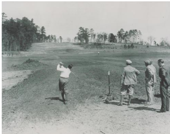
Jones driving off a crude tee during construction of AN on what is now the par 5 570-yard uphill No. 8 hole. Mac stands next to him in his plus fours and Hogan hat.
