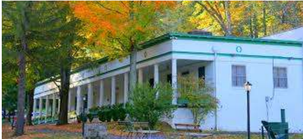
The Meeting House, site of Capon's theater and other facilities
